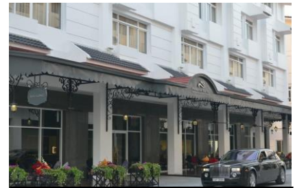
PARADISE SUITES HOTEL, HALONG BAY
